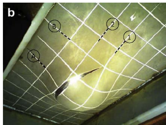
Fig. 20. Deformation and the fracture pattern of the unstiffened plate [1].
